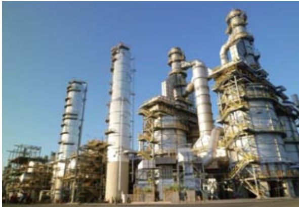
Hyundai Cosmo Petrochemical Co., Ltd. para-xylene (PX) production unit
