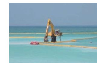
Installation of silt curtains
