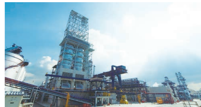
Sakai Refinery coker
