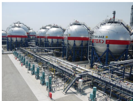
LPG tanks newly installed at Chiba Refinery
