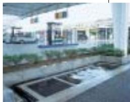
Oil-water separation unit, where oil is removed from water and water pollution prevented
