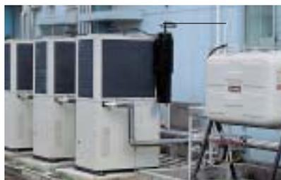
Kerosene heat-pump air-conditioning unit<sup>2</sup>
