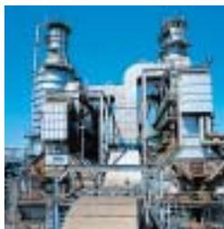
Fuel Gas Denitration unit which removes NOx from exhaust gases
