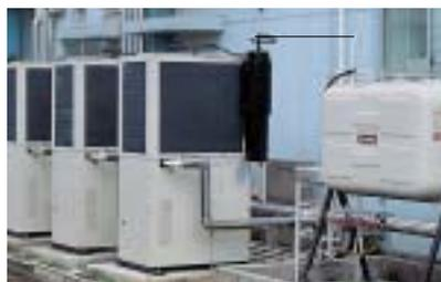
Kerosene heat-pump air-conditioning unit<sup>2</sup>
